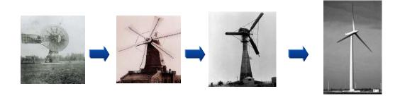
The cost per kilowatt hour (kWh) of electricity dropped by about 50 per cent with the appearance of this generation of wind turbines. Over the period of 130 years (reference Nicolas, Iñigo Martija de. Wind Energy Evolution And Expectations provides an excellent detailed description of these developments) the designs evolved from a complicated wooden flat panel design to a quais-3d aerodynamic design with three blades producing 9 times the energy for the same weight.
